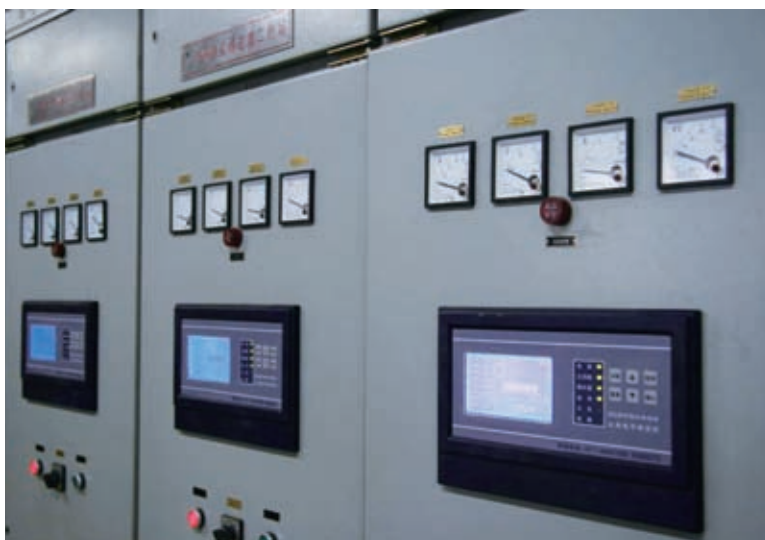
De-dusting high pressure control case following the upgrade of Dianta Power Plant of Shendong Power.
