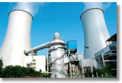
Smoke-tower combination technology equipped with desulphurization facilities applied in Sanhe Power Plant
